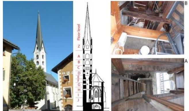
Figure 25. From left: San Luzi Church with Bell tower; cross section of the tower with its floors; view of inside from A and B floors
