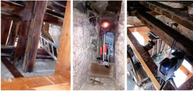
Figure 28. Bell tower inside. From left: View from the A-floor to the Z floor; prism number 1004; scan between the A and Z floor
